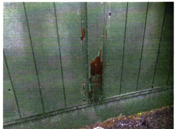
Exposed Wood with Dry Rot
